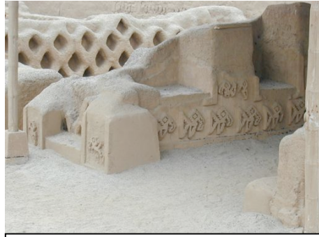
Fig. 04 - Tsudi Palace, Chan Chan, Peru. Protection layer on the top of the walls.
