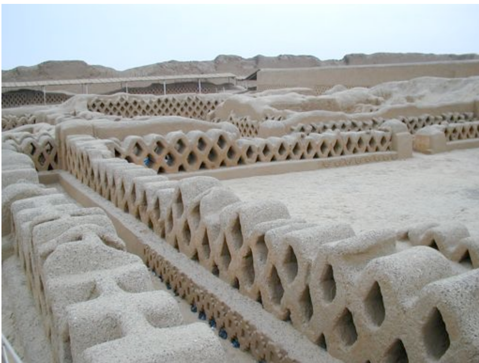
Fig. 02 – Tschudi Palacio, Chan Chan, Peru. Know-how of the adobe constructive technique.
