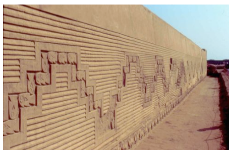
Fig. 01 - Tschudi Palacio, Chan Chan, Peru. Repair of the lacunas with reconstruction of architectonic surfaces.
