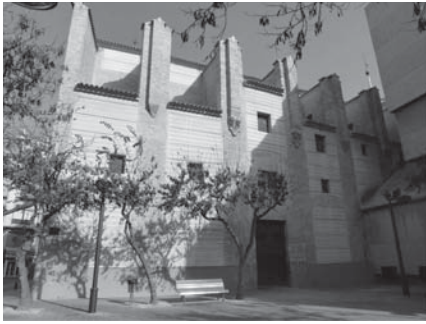
Figure 11. South façade of the Church of La Merced (Murcia) (Vegas & Mileto).
