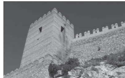
Figure 10. South wall of the Islamic castle at Almería (Spain) (Vegas & Mileto).
