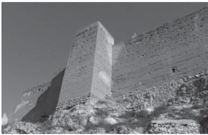
Figure 12. Restored wall of Jorquera (Albacete, Spain) (Vegas & Mileto).
