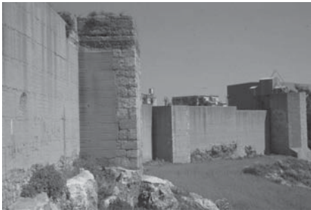
Figure 6. General view of the Niebla city walls after restoration (Huelva, Spain) (Vegas & Mileto).
